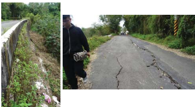
Southern Taiwan Earthquake of February 6, 2016
