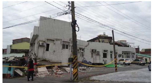
Southern Taiwan Earthquake of February 6, 2016
